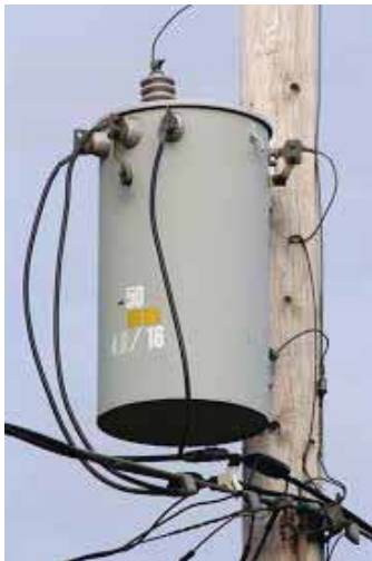
Pole Mount Tx Refurbs
