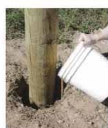
Pour mixture into prepared hole with pole
